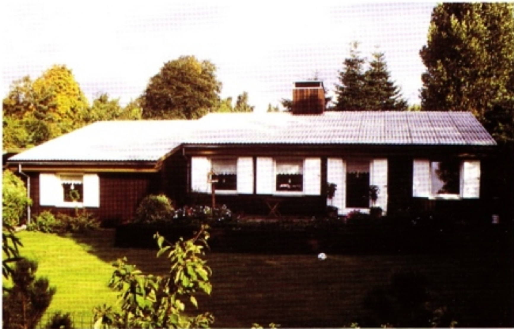
Most of the windows are located on the south side of the house, to maximise the collection of solar gains.
